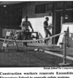
Construction workers renovate Escondido Elementary School to upgrade safety systems.
