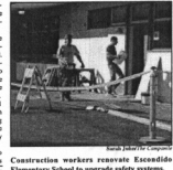
Construction workers renovate Escondido Elementary School to upgrade safety systems.
